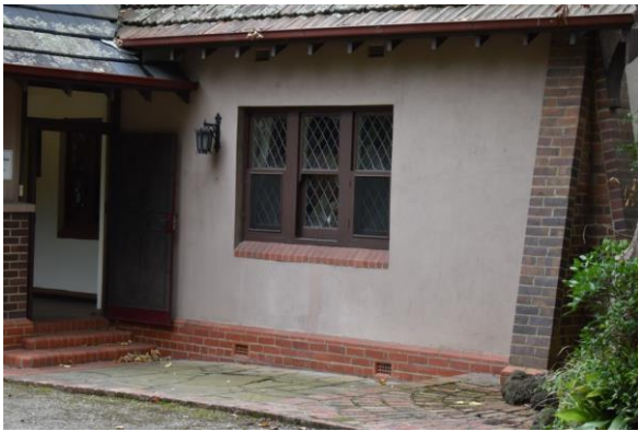
Detail view of ground floor fenestration, brick window sill, and clinker brick corner buttress (source: Extent Heritage Pty Ltd, 2022).
