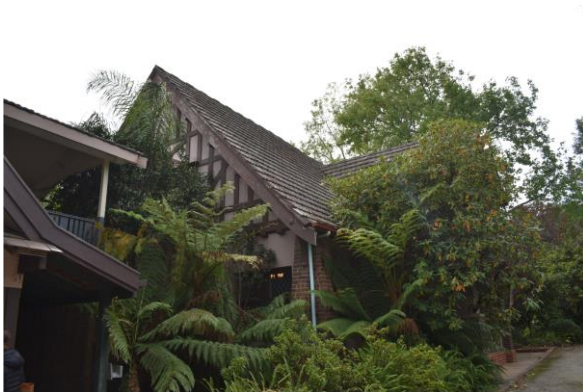
North-east facing view of main residence (source: Extent Heritage Pty Ltd, 2022).
