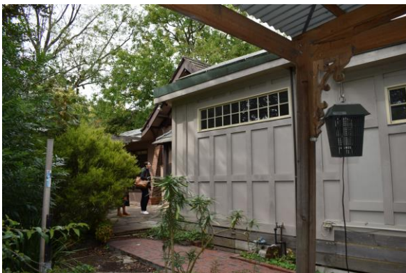
North-east facing view of 1996 rear addition (source: Extent Heritage Pty Ltd, 2022).
