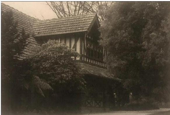
Black and white photograph of Alta Dena entrance portico and upper storey gable projection, date unknown (source: Unknown, n.d. View of Alta Dena. Black and white photograph. Unknown collection. Lilydale & District Historical Society).
